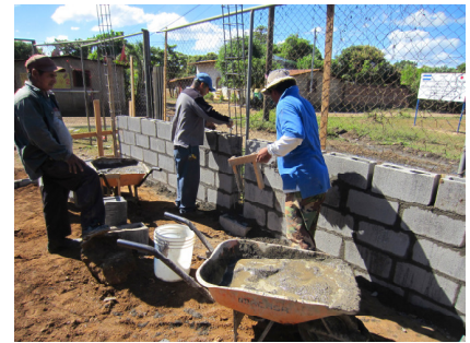
Andrés Hernández, our "maestro de obra" hired construction workers from the community and supervised family volunteers. The work was hard; the energy was respectful, positive and fun.
